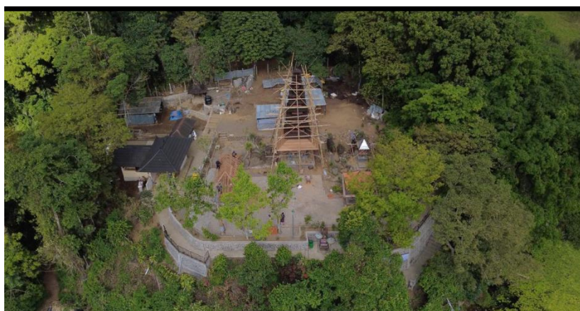
Figure 1. Pura Dalem Tamblingan during the renovation process (Source: Personal documentation, 2025)
